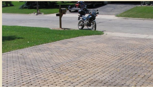
Alternative pavers such as those used in this residential driveway can help to reduce heat gain and keep stormwater runoff on-site.
