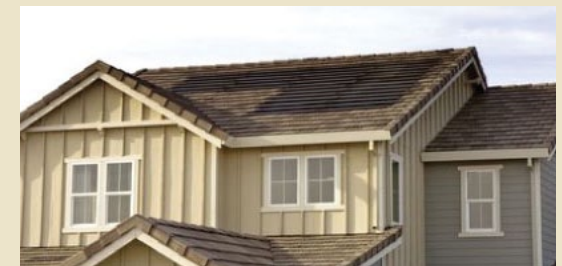
Energy efficient design could include such features as solar roofing tiles, which are combined with conventional roofing in this home.
