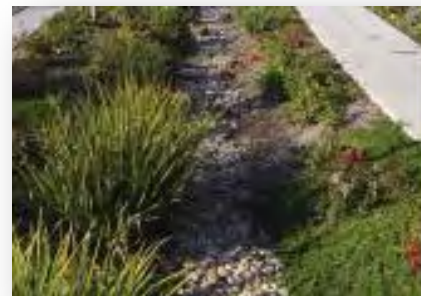
Typical bio-swale surface water filtration in a landscaped area.
