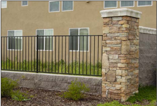
Example of open fencing with masonry knee wall and stone pilaster.
