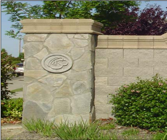
Example of masonry wall
